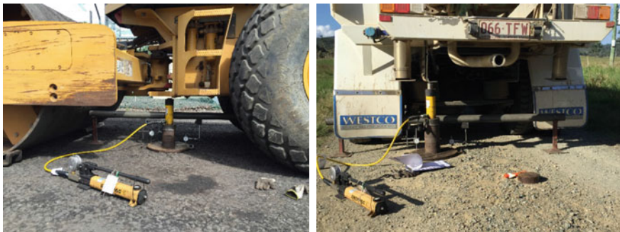
(a) Static Plate test on previously constructed road
