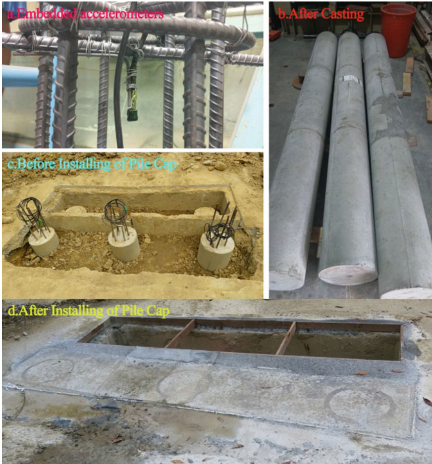
Fig. 4. Photographs taken during the construction of three model piles
