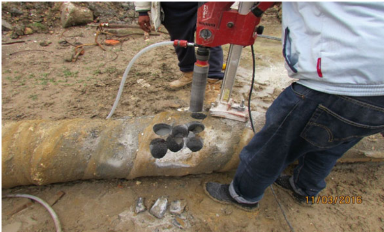
Fig. 3. Coring concrete samples of the uplifted RIT pile ( L = 6 m, D = 0.4 m, Essalema City, Tunis)
