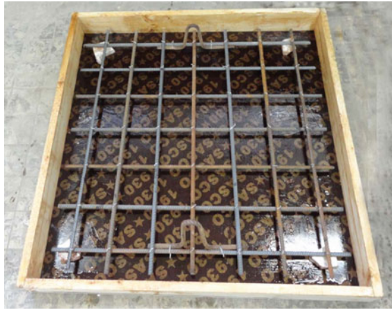
Fig. 2. Reinforcement and mold
